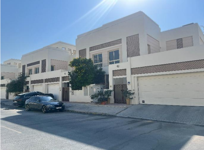
Source: JLL Inspection 2025
