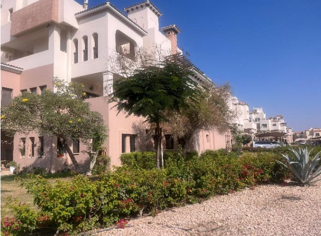
Source: JLL Inspection 2025
