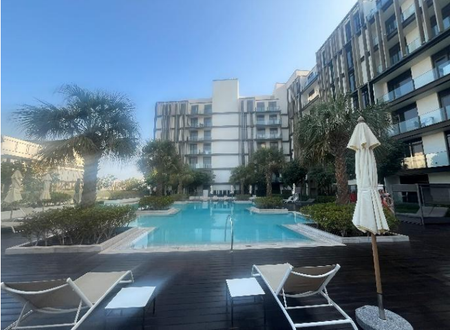
Source: JLL Inspection 2025
