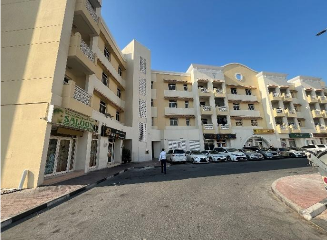
Source: JLL Inspection 2025
