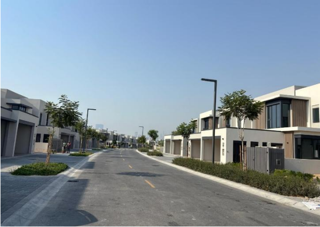
Source: JLL Inspection
