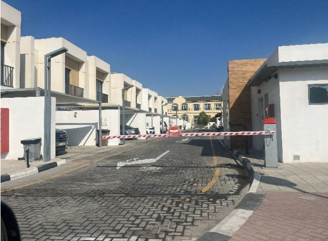
Source: JLL Inspection 2025
