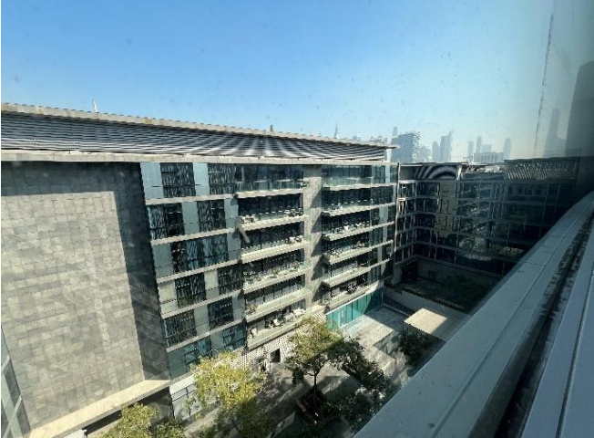
Source: JLL Inspection 2025
